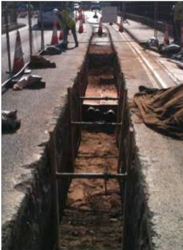
FIGURE 16 TRENCH DUCTS BEING BACKFILLED WITHIN THE CARRIAGEWAY - DUCT BLOCK CAST, BACKFILL CABLE COVERS, AND PARTIAL BACKFILL (consent from Neary Construction).
