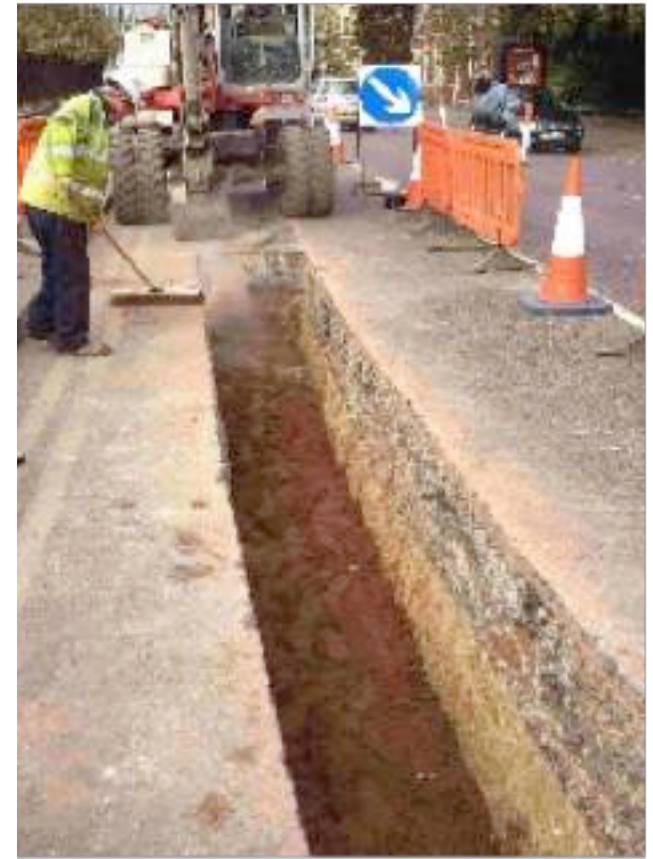
FIGURE 16 TRENCH DUCTS BEING BACKFILLED WITHIN THE CARRIAGEWAY - DUCT BLOCK CAST, BACKFILL CABLE COVERS, AND PARTIAL BACKFILL (consent from Neary Construction).
