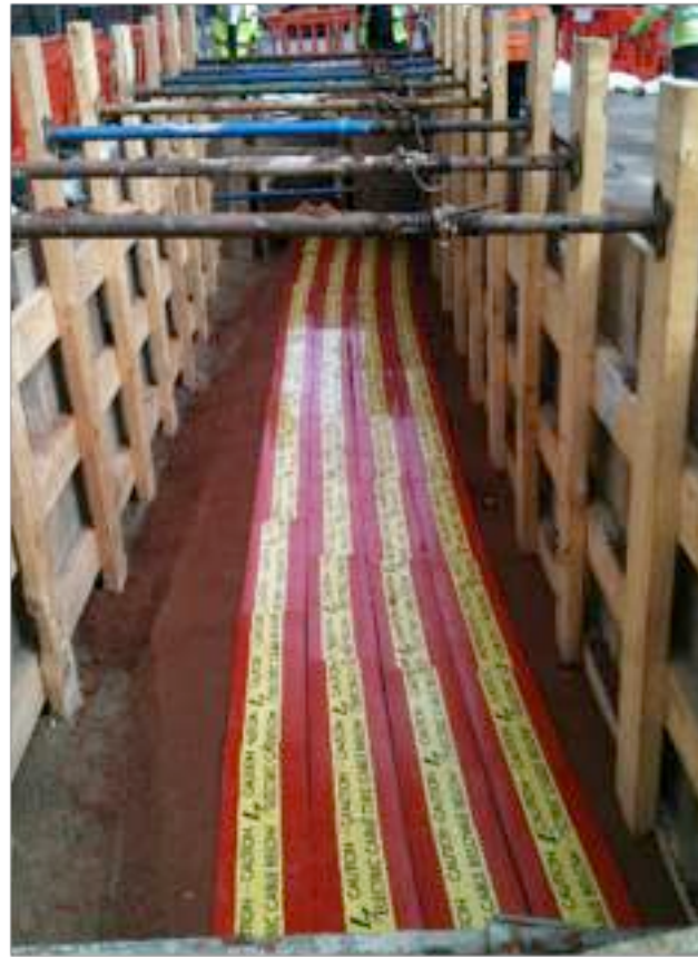
FIGURE 16 TRENCH DUCTS BEING BACKFILLED WITHIN THE CARRIAGEWAY - DUCT BLOCK CAST, BACKFILL CABLE COVERS, AND PARTIAL BACKFILL (consent from Neary Construction).
